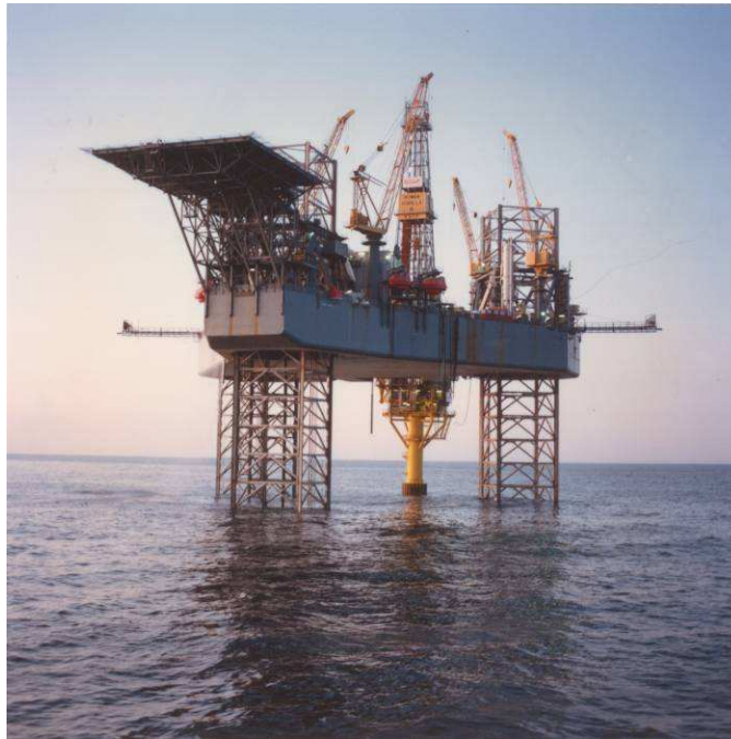
Figure 2-12. Typical Jack up Drilling Rig (Rowan Gorilla III) -(Courtesy of Rowan Companies Inc)
