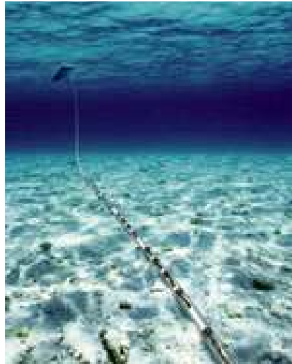
Figure 2-8.b) Schematic of a cables laying on seafloor. Typical diameter 3.8 cm-7.6 cm (1.5in-3in) - Courtesy of Sonardyne.co.uk).
